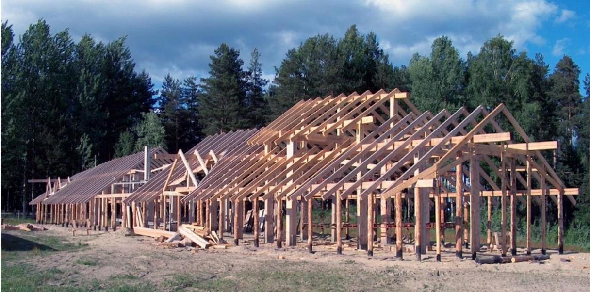
**Figure 2.** Photograph taken in 2003 during reconstruction of the large hall at Veien, Ringerike, Buskerud.
