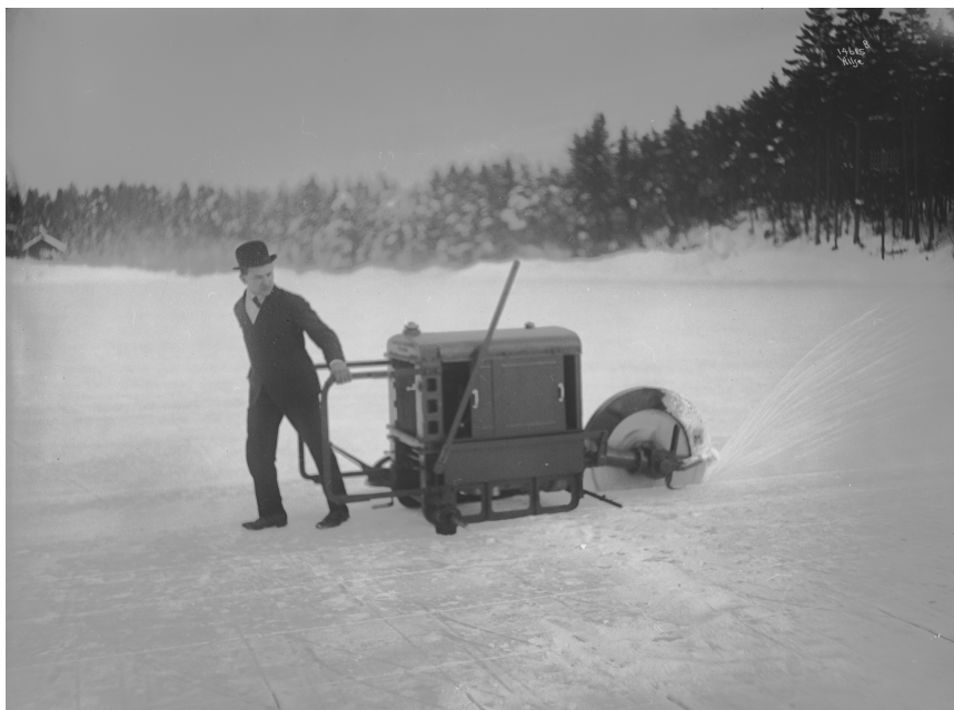
Figure 8.3. Machine-cutting of Norwegian lake ice in 1921, a means of reducing the costs of harvesting when wage costs were rising (Norsk Folkemuseum NF.WB 14615).
