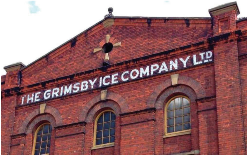
Figure 5.3. The Grimsby Co-operative Ice Company's factory stands to this day, but operations ceased in 1990. The complex is a listed building, and it was once the largest ice factory in the world (Wikipedia - CC BY-SA 2.0).
