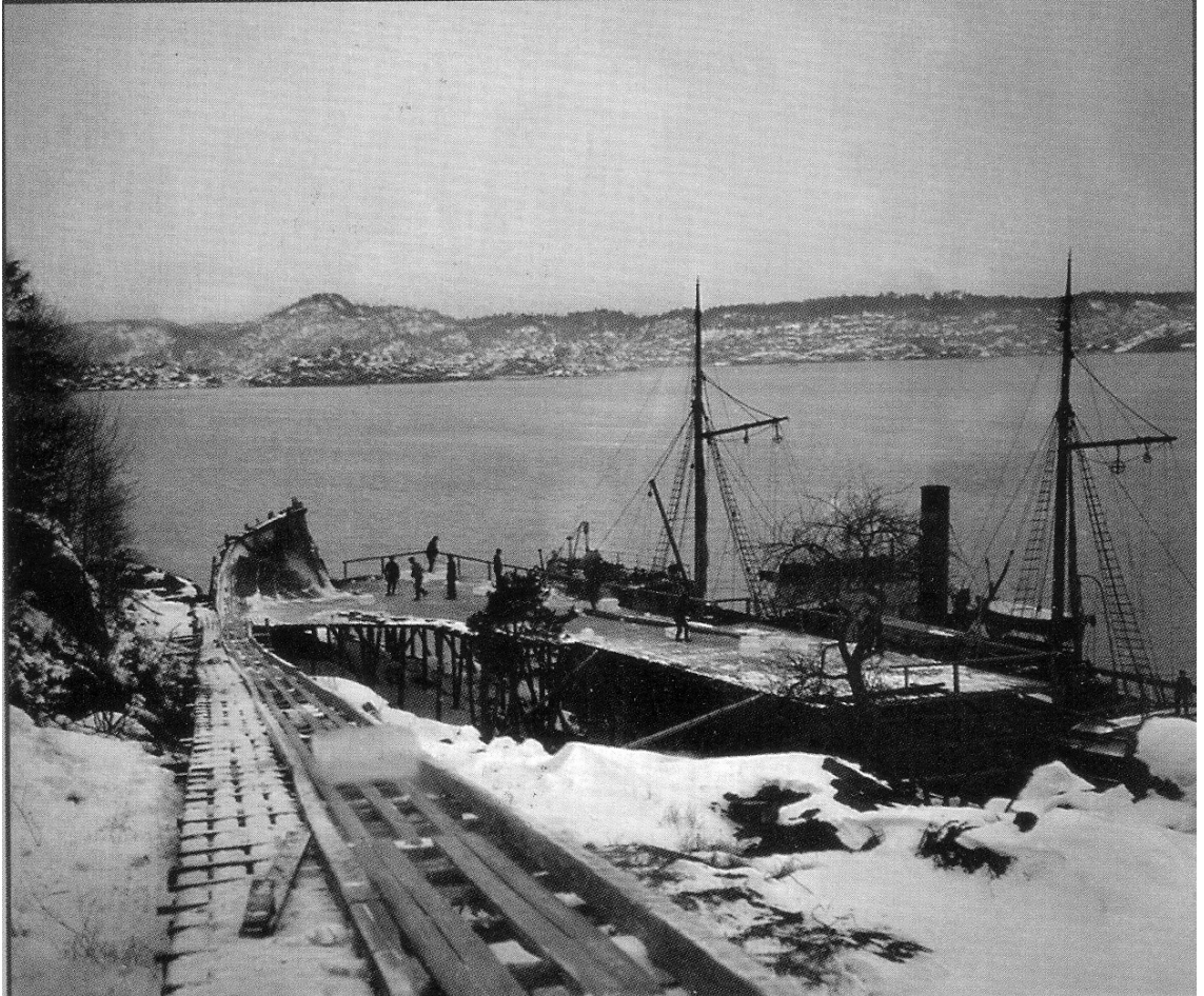
Figure 2.10. An ice block on a wooden switch-back railway near Kragerø as it approaches the shoreline, ice workers and ice-steamer awaiting loading (Berg-Kragerø Museum, Creative Commons BY-ND 4.0).
